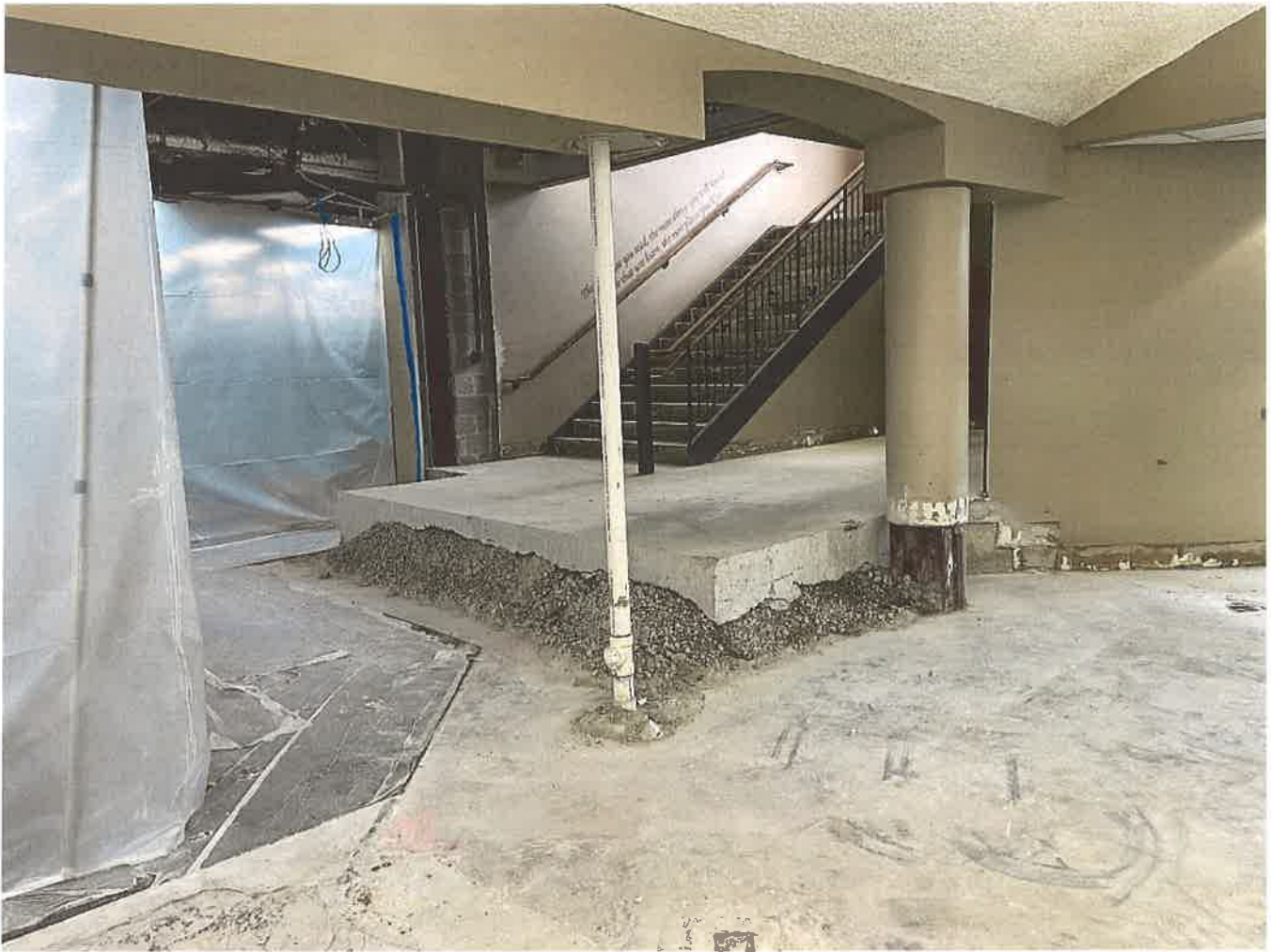
Bottom of stairs demolished
